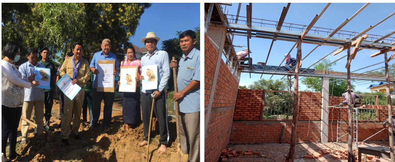
New school building: Constructing additional classrooms for the extracurricular program in Rong Vean
