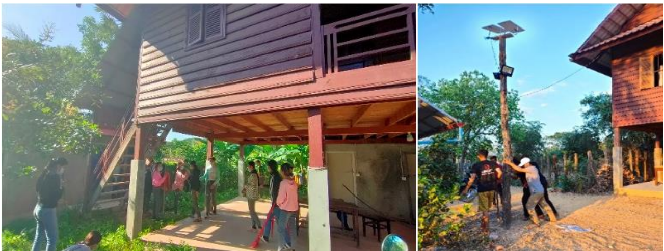
Boarding Me: Clean up and refurbish, let lighting up!
